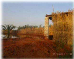
**Picture 3:** "Za'rb" a tree leaf wall between two orchards
