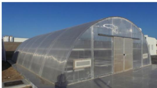
**Fig. 1.** Polycarbonate Drying House (PDH)
